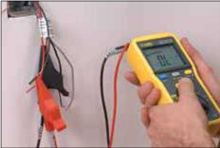
**4** Once the tile installation is complete, retest the heating cable and record values in the heating cable tests log (page 39).
