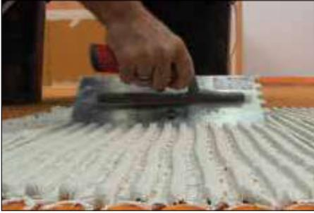
**1** Tile can be installed over DITRA-HEAT and DITRA-HEAT-DUO immediately; no need to wait for the mortar to cure. Fill the matting with SET, ALL-SET, FAST-SET, or unmodified thin-set mortar and comb additional mortar over the matting using a trowel that is appropriate for the size of the tile.
