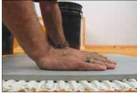
**2** Solidly embed the tiles in the setting material, sliding the tile back and forth perpendicular to the tile ridges underneath. This will help collapse the mortar ridges and improve contact between the mortar and the tile. Make sure to observe the open time of the bonding mortar. If the mortar skins over prior to tile installation, remove and reapply.
