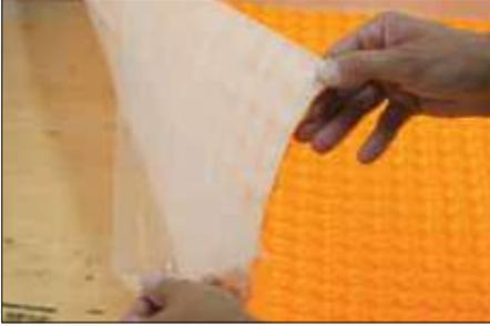
**1** Remove release liner from DITRA-HEAT-PS / DITRA-HEAT-DUO-PS membrane.
