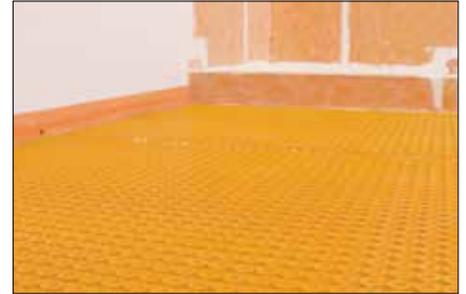
**3** Abut adjacent sheets and align the studs on the top of the matting to make subsequent heating cable installation easier.
