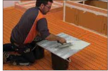
**3** Periodically remove and check a tile to ensure that full coverage is being attained.
